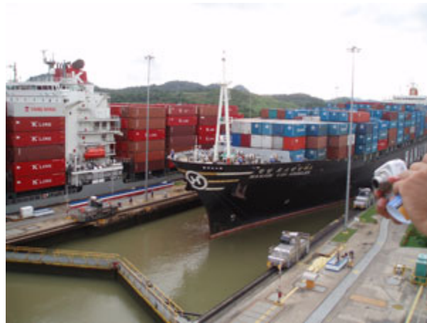
Cargo ship on the Panama Canal
